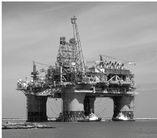
Photo Courtesy of BP © Press Images: Thunder Horse Oil Platform (image highlights the location of a typical pipeline welding job)
